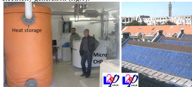
Fig. 1. Micro CHP and 17kW PV panels at L2EP laboratory
