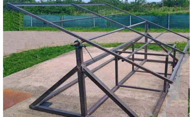
Fig. 3 Picture of the constructed structure
