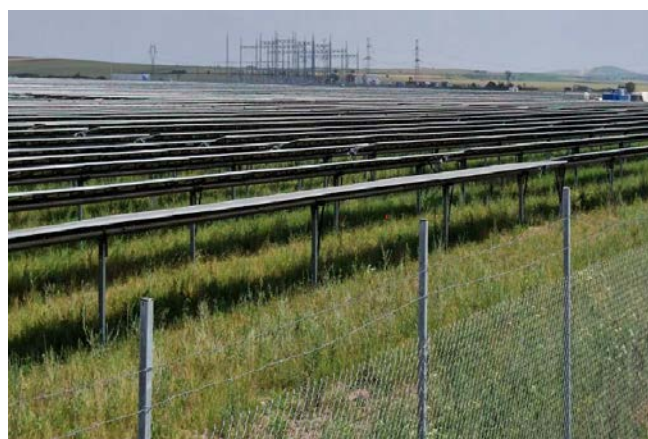
Fig. 2 Orientation of the panels to the east, slope below 20^\circ
