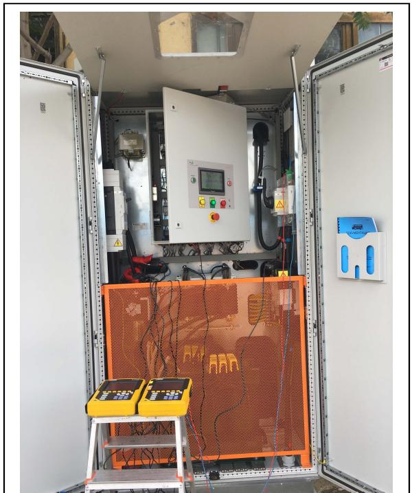
Fig. 2. Connection to a CS with two energy analysers.
