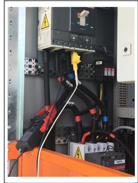
Fig. 6. Upstream DC Connection to CS.
