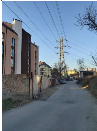
Fig. 1. A snapshot of the investigated building and line
