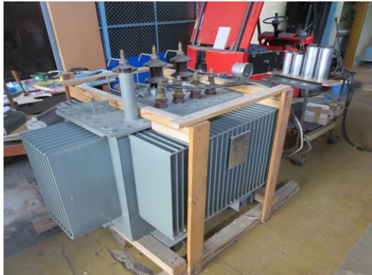
Figure 3. Type of appearance of transformer used in experimental investigations: type ETB 400-10/0.4, voltage 10000/400V, current 23.09/577.4 A, f = 50 Hz, 3-phase step-down transformer.
