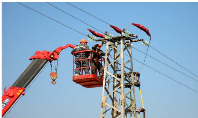
Fig. 5. Installation of protective equipment against birds
