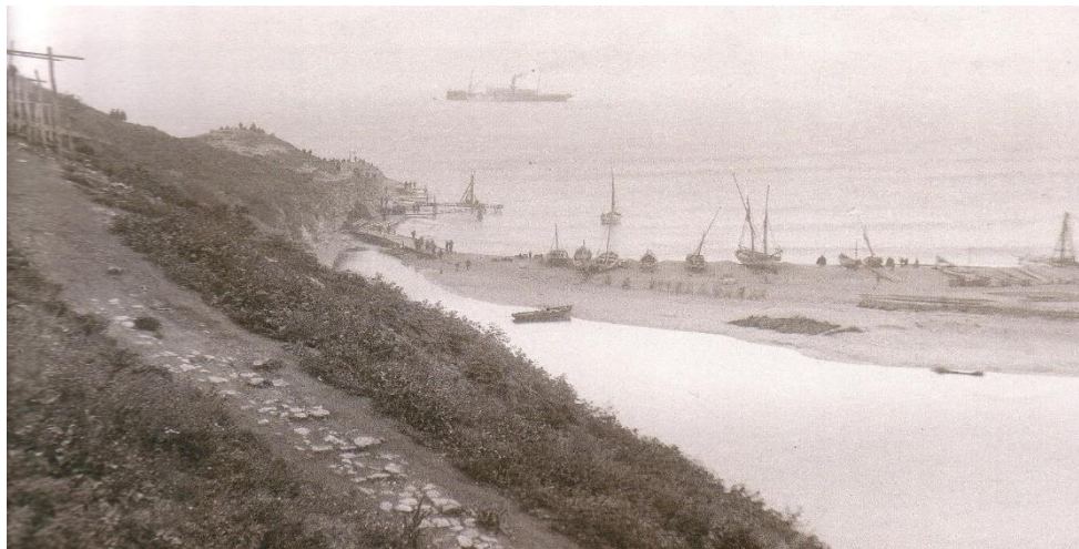
Fig. 1: The outline of Cape Varna in the late nineteenth century and sands separating the bay of Varna lake. Today Cape Varna does not exist, in its place was built the new port of Varna
