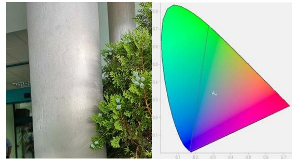
Fig. 5 a) Metal coating of the columns at the entrance of the building b) color coordinates of the columns at CIE xyY color space
