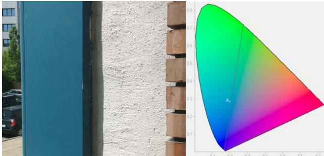
Fig. 4 a) Metal coating of the edges of the building and window frames, b) color coordinates of the coating in CIE xyY colour space
