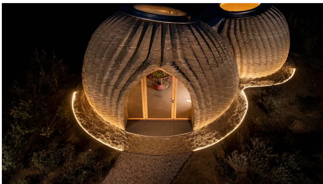
Fig.4 One of the first 3D-printed buildings, located in Milan, Italy, designed by Mario Cucinella Architects
