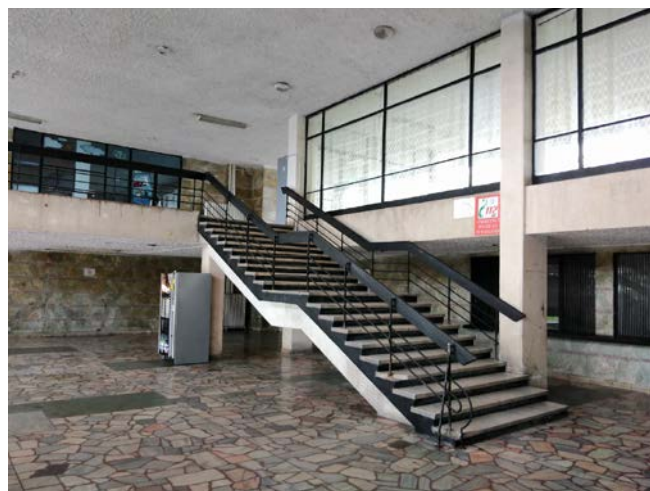
Fig. 1. Condition of the lighting installation in the railway station.
