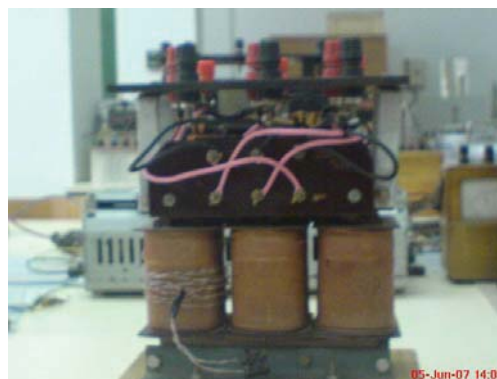
Fig.1. Front view of the transformer
