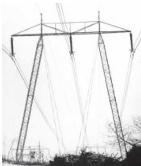
Fig.1. 2x400 kV three-phase power line.
